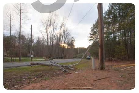
Don't go close to water that is near a downed wire. Puddles, streams, and other bodies of water can become energized. Be careful after storms around streams or other sources of water in case a wire has fallen in them.
