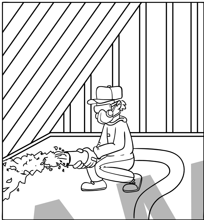
Installing Insulation
