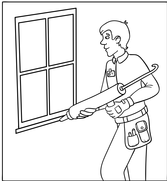
Caulking Cracks
